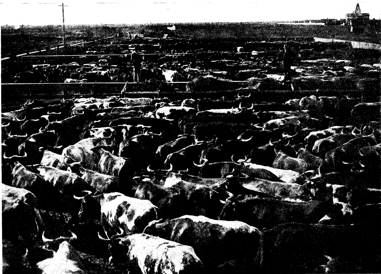
Section of C.P.R. Stock Yards, Winnipeg. In 1906 a Winnipeg firm of live stock exporters led the world. The present yards are being extended and plans are under way for a big union stock yards that will give adequate room for the increasing trade. Winnipeg has four abattoirs with a total killing capacity exceeding 5000 head of stock per day.
